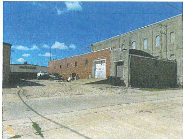
Existing building from back parking area looking southwest.
