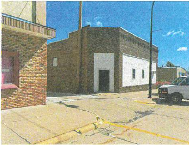
Existing building from E State St looking northeast.
