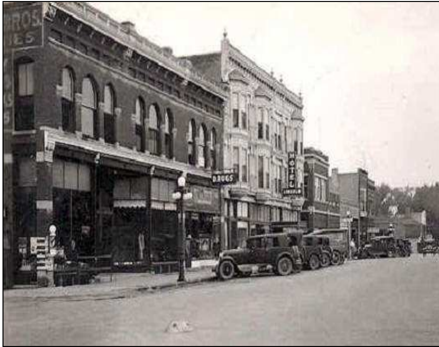
Figure 15: Lincoln Way, view southwest, ca. 1917, the entire frontage is “fireproof, note the traffic bump in the street intersection http://jeffersoniowanews.com/News/photoarchives.htm
