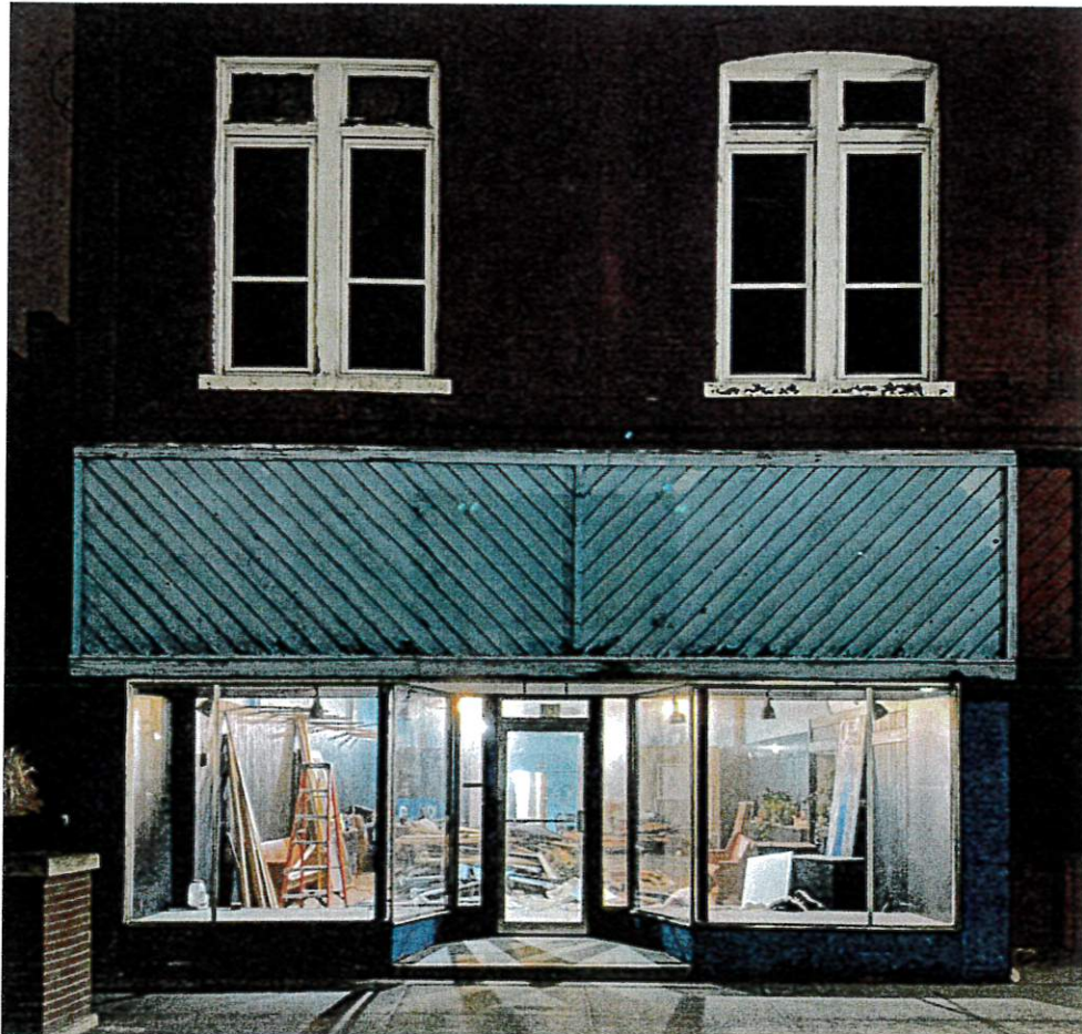
Inside during deconstruction and removal of debris and junk.
