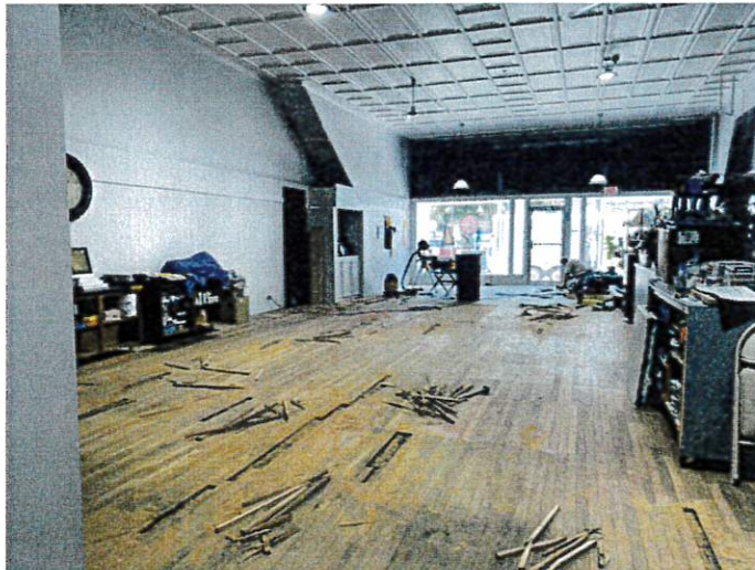
Floor was restored.
