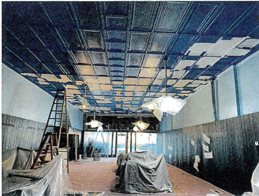
Original tiles were painted a brighter color, as we were unable to remove the blue.
