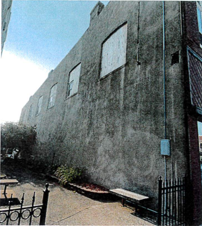
South Side after powder blasting to remove graffiti
