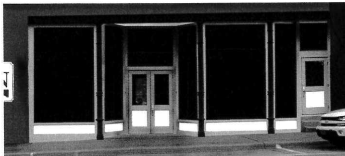
Storefront Transom Window Layout Under Awning
